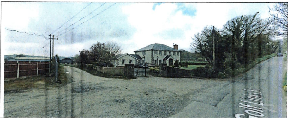
Figure 3: Photo of the dwelling shown on the aerial photo at Figure 2 taken from google street view. As can be seen road shown on the righthand side of photo the Golf Links Road rises to a humpback bridge which traverses the nearby railway line.
