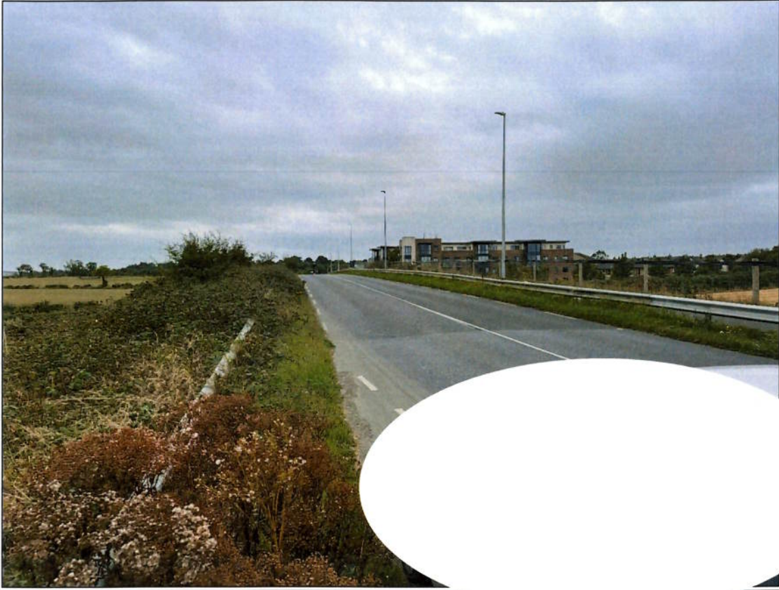
View towards proposed substation at Colpe Road, Southern Environs of Drogheda along L-1611-0
