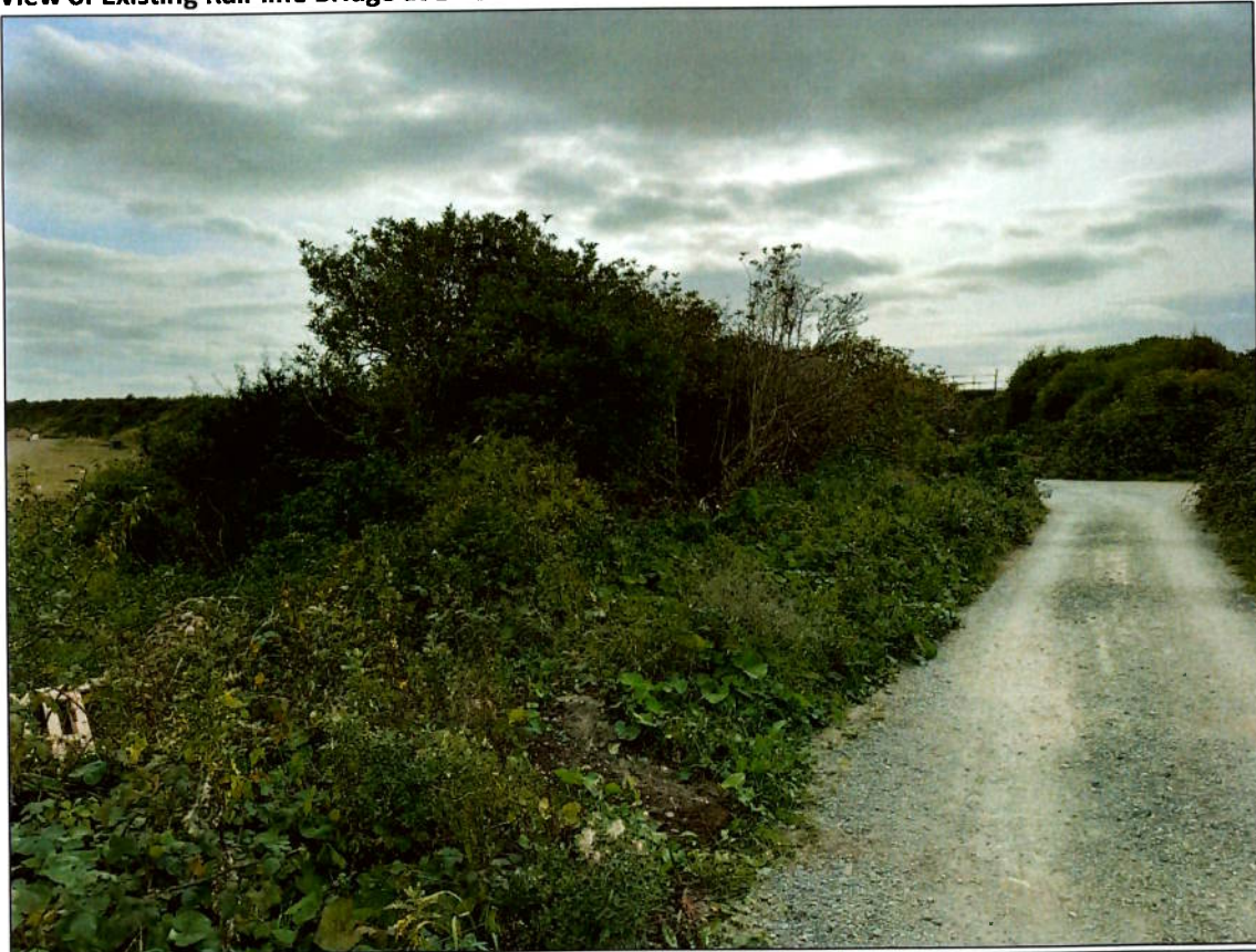
View of Existing Rail-line Bridge at L-16163-0
