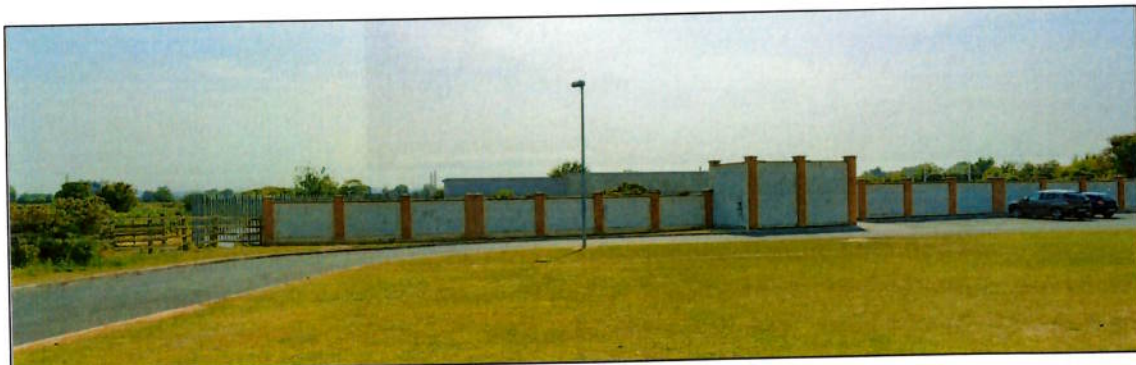
Fig. 4: Proposed Substation at Objective 1 (Bettystown Zoning Map) - Photomontage (Vol. 3B EIAR, p.36)
