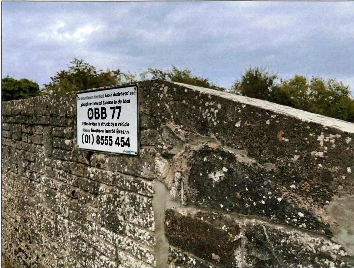
L-16115-0 Bridge over Rail line (Between Pilltown Road and Colp)
