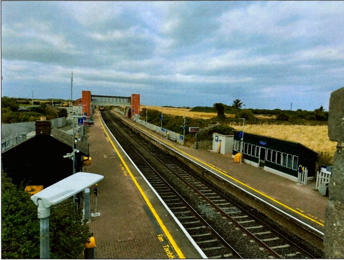
View from Overbridge at Existing Gormanston Train Station
