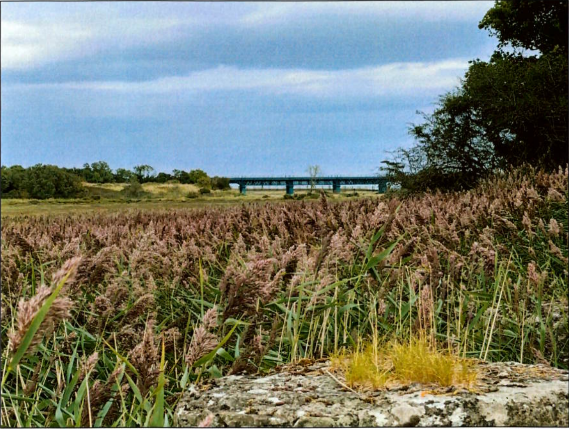
View of Existing Laytown Viaduct from L-16161-12
