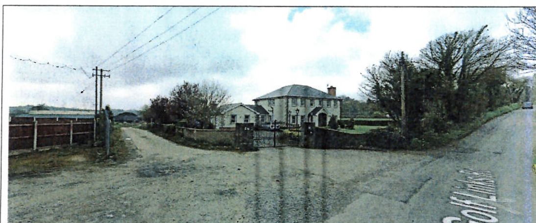
Figure 3: Photo of the dwelling shown on the aerial photo at Figure 2 taken from google street view. As can be seen road shown on the righthand side of photo the Golf Links Road rises to a humpback bridge which traverses the nearby railway line.
