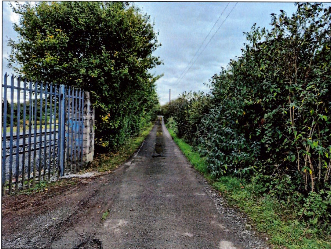
Figure 1.4: Existing McGrath's Lane (East) Looking West toward Bridge
