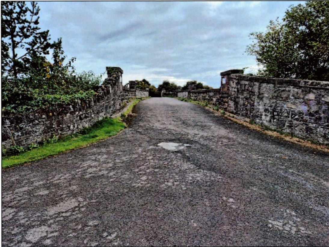
Figure 1.3: Existing Overbridge – Looking South
