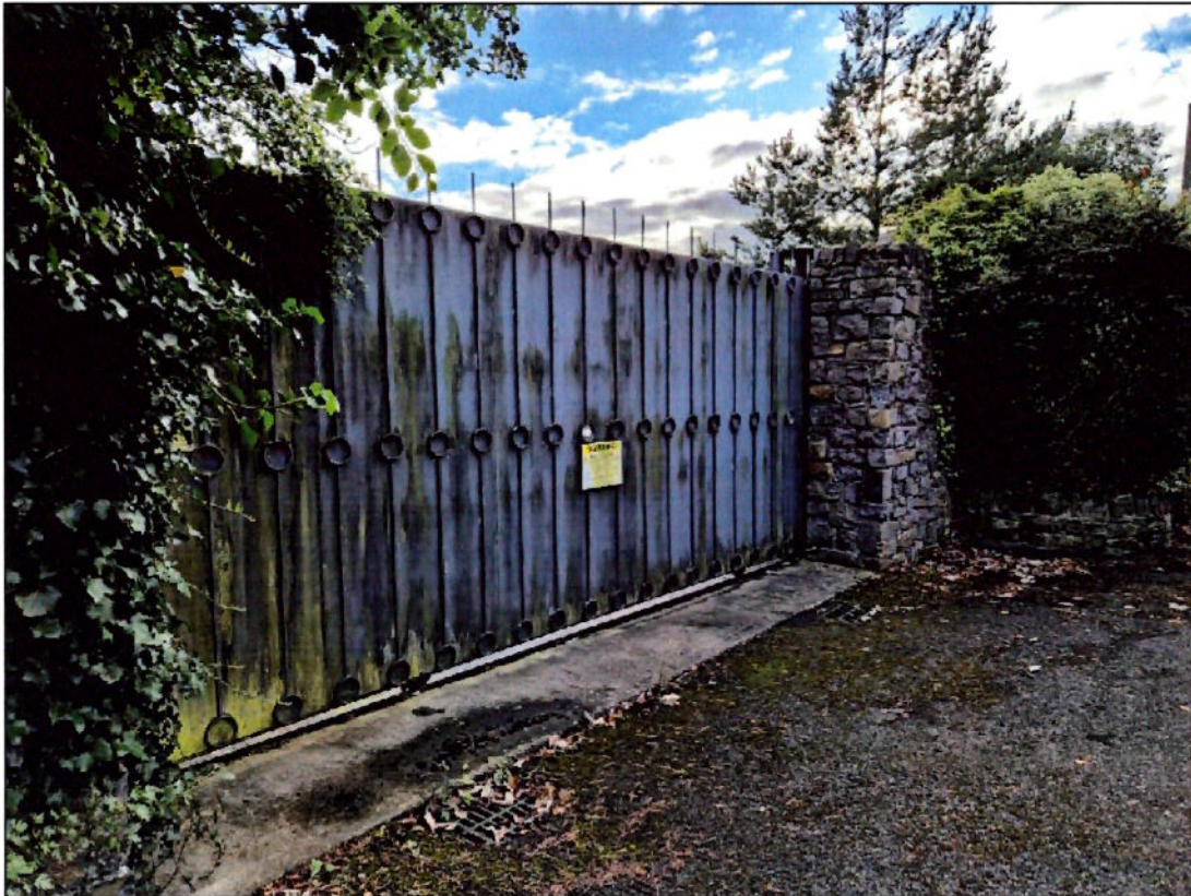
Figure 1.6: Existing Rail Yard Emergency Access off Access to Mc Grath's Lane
