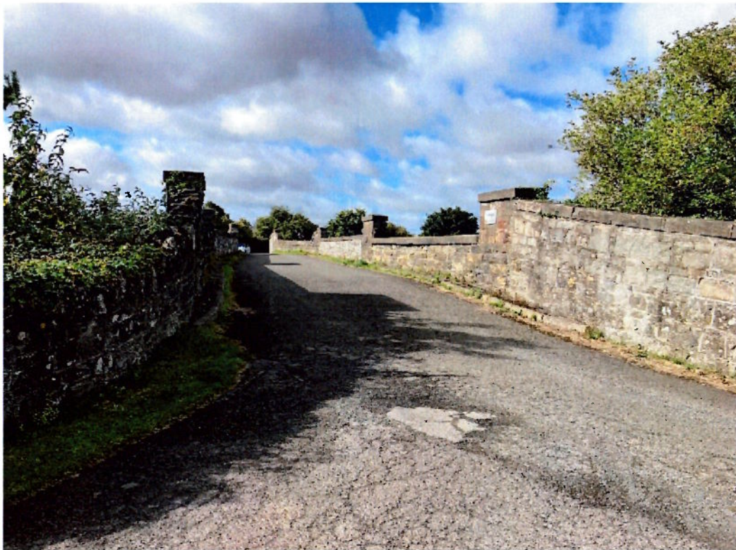
Figure 11: Appearance of Railway Terrace bridge looking south
