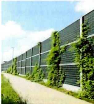
External Sound Barrier wall
