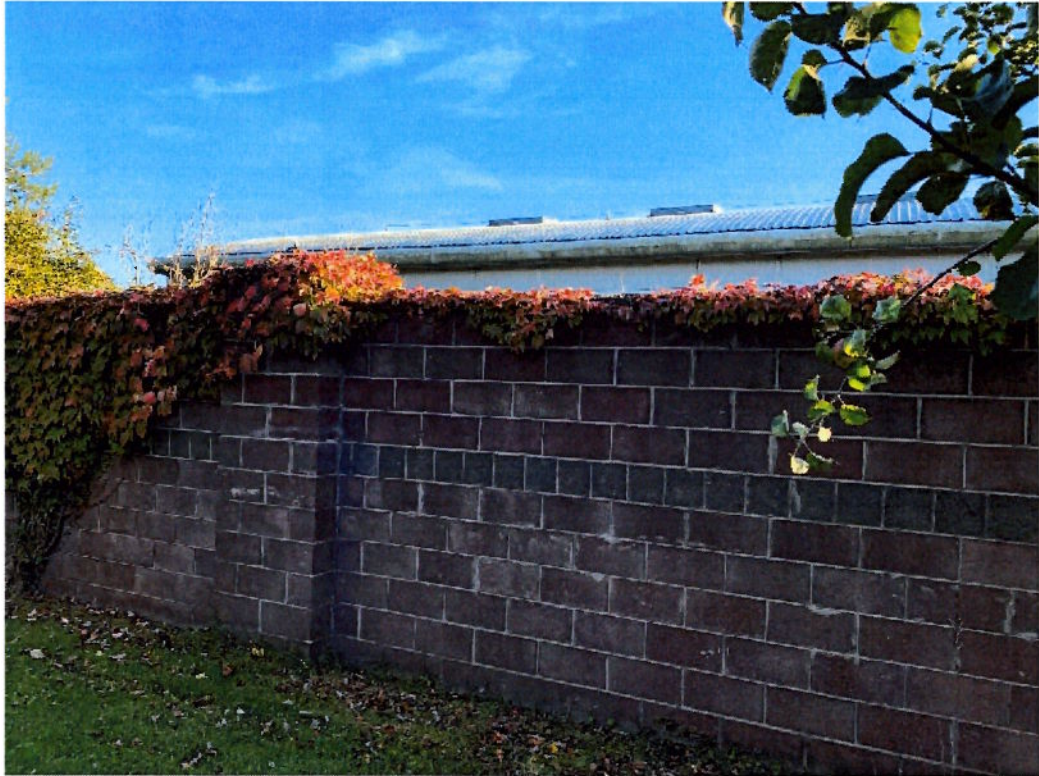
Figure 10: Existing block wall at Chanticleer
