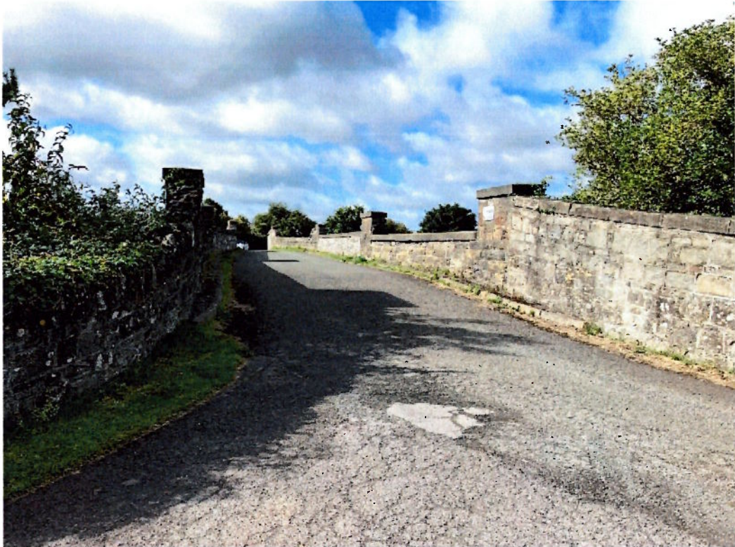
Figure 14: Appearance of Railway Terrace bridge looking south
