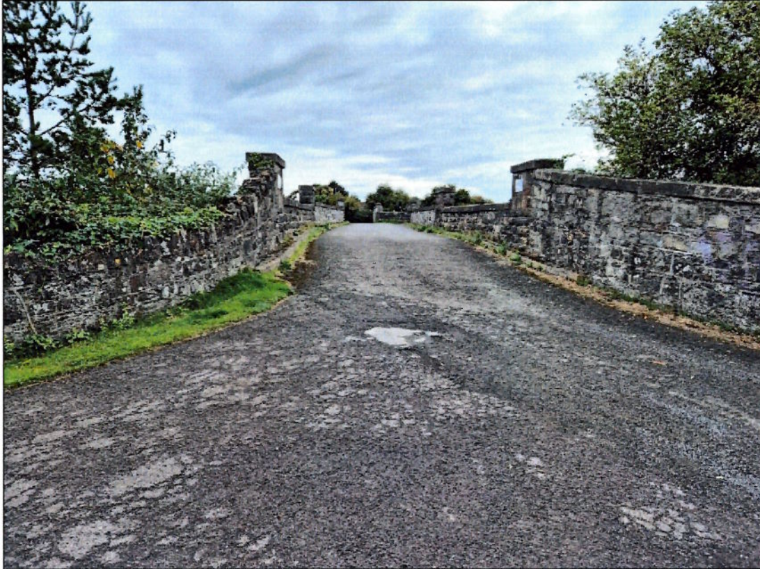
Figure 1.3: Existing Overbridge – Looking South
