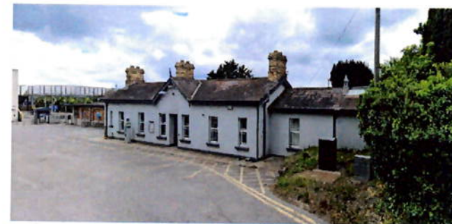
Rush & Lusk train station building on east side of railway
